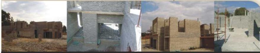
PICTURES LEFT: The Spa under construction
