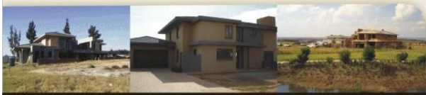
PRIVATE PICTURES LEFT: A few of the private residences under construction
