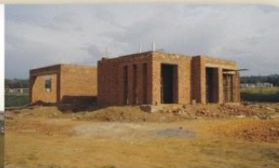
PRIVATE PICTURES LEFT: A few of the private residences under construction
